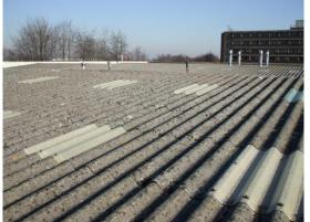
Example of fragile fibre cement sheeting where special precautions would be needed prior to commencing work.
